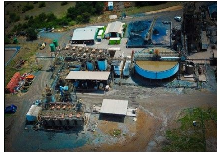
Above: Doornbosch Secondary Flotation Circuit (old Steelpoort PGM plant relocated) Below: Doornbosch Secondary Flotation circuit
