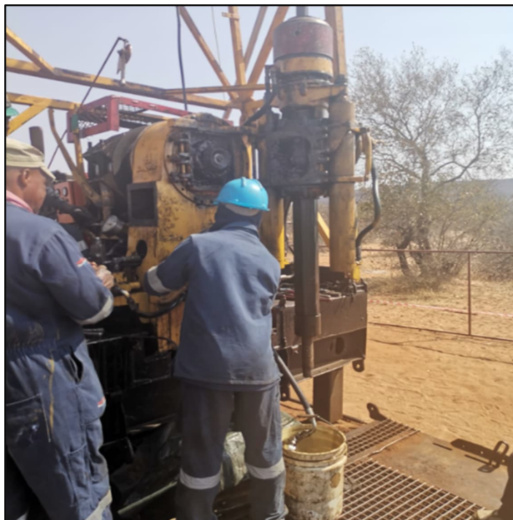
Figure 23. Rig 5 during gearbox repairs.
