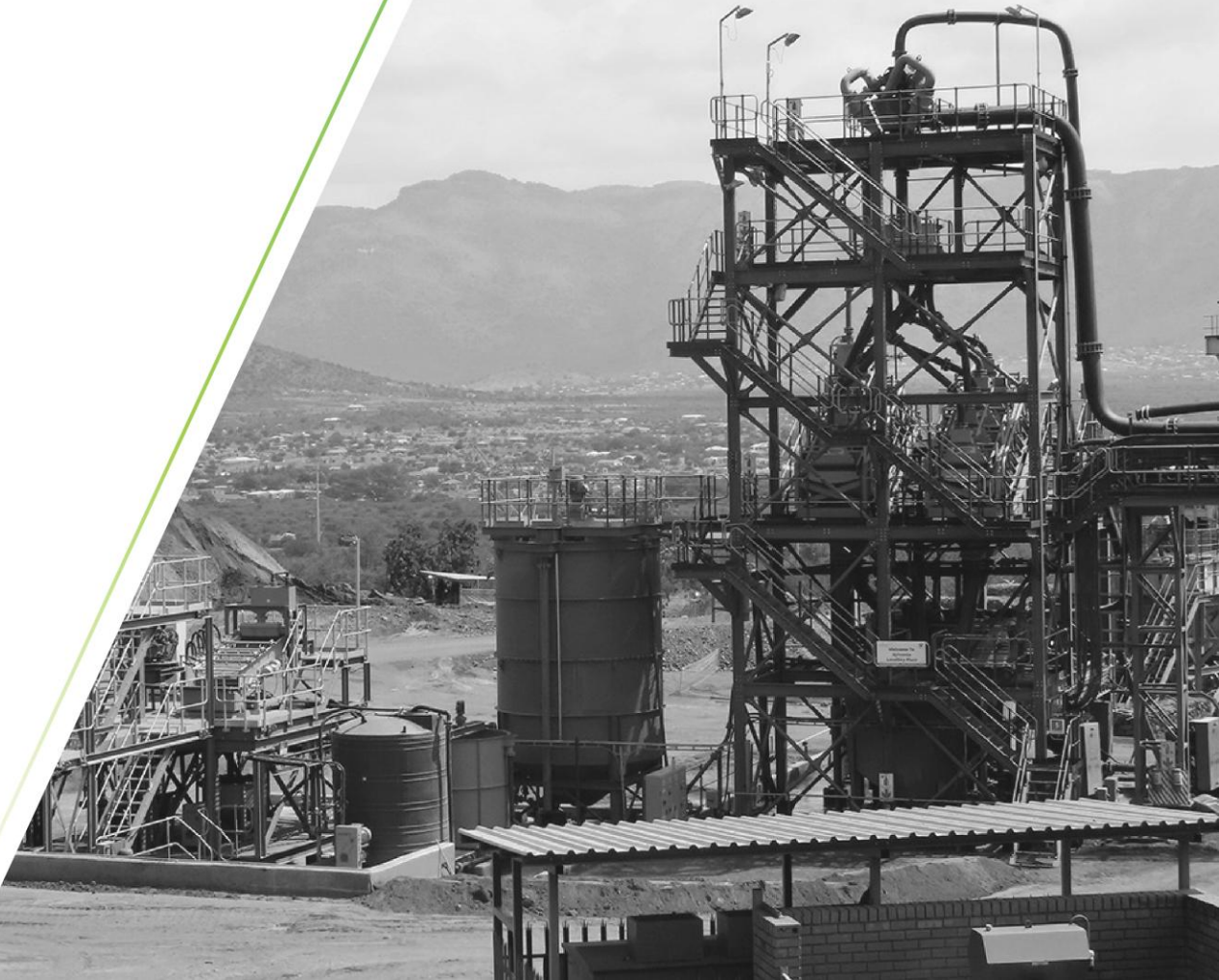
Lannex Fine Screening Circuit
