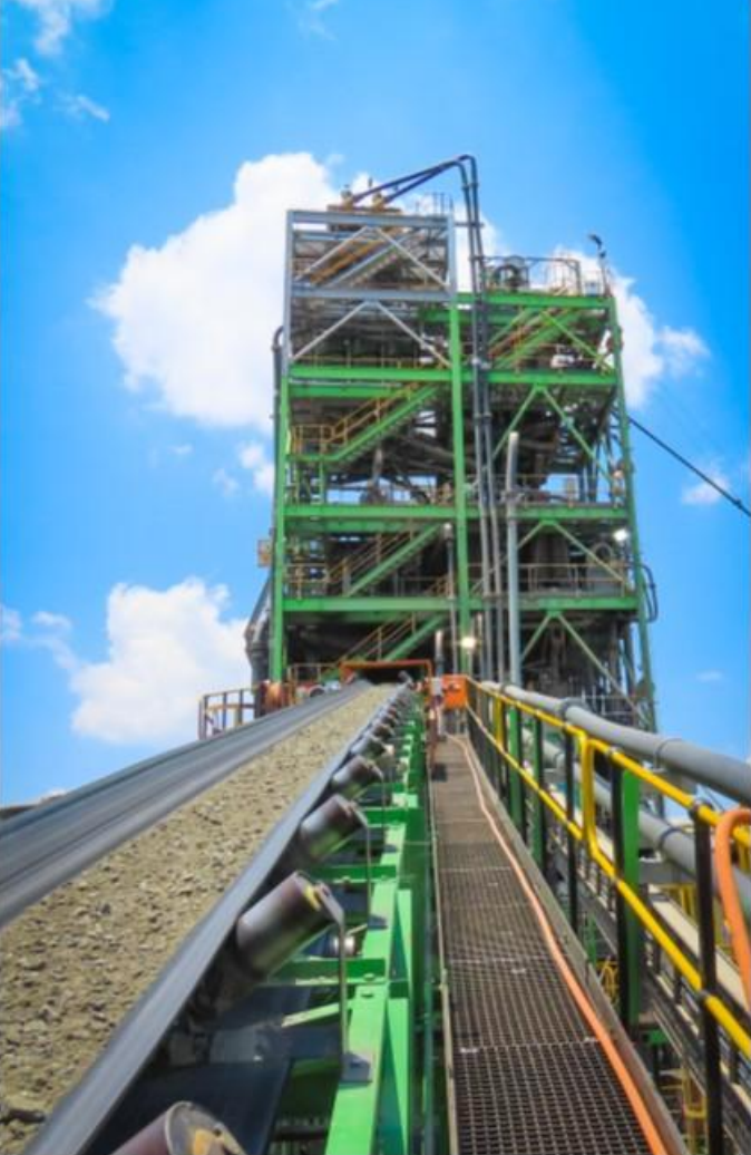
Mill Feed Conveyor and Primary Chrome Spirals
